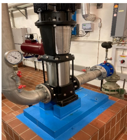
Rentvandspumpe
